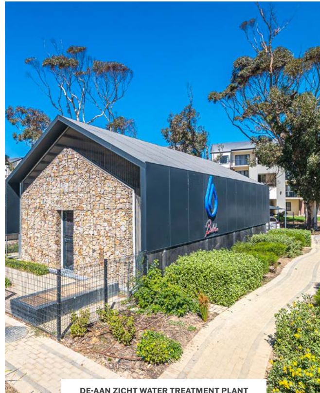
DE-AAN ZICHT WATER TREATMENT PLANT
