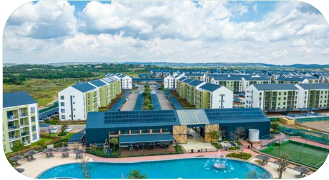
GREENCREEK® HAZELDEAN - TSHWANE
